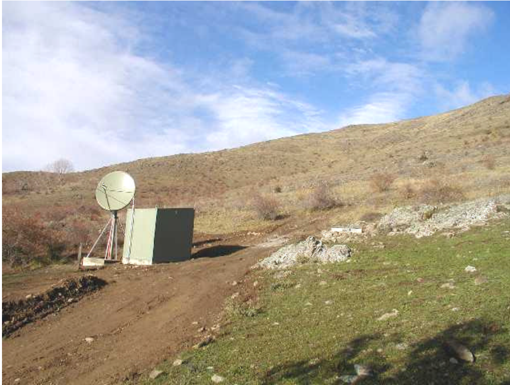
Figure 2. Photograph of a NZNSN station showing the VSAT dish (left) and equipment hut, with the top of the sensor vault just visible on the top of the rock outcrop to the right.
